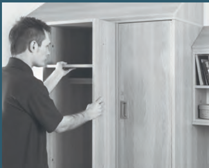
Furniture modules can be removed for repair while the rest remains in situ.
